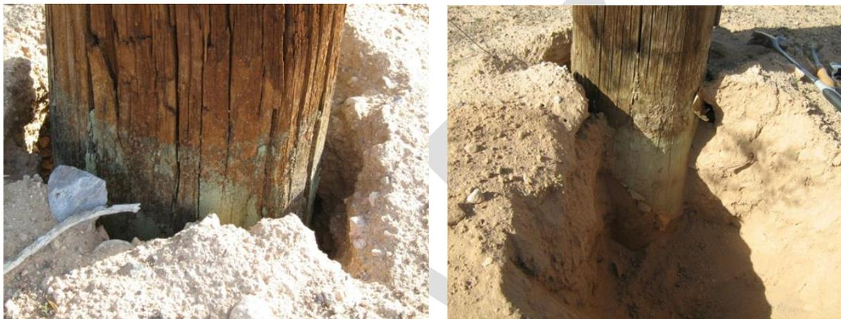
*Figure IV-1. Poles in the APS system after excavation showing evidence of animal gnawing on the barrier bandage.*
