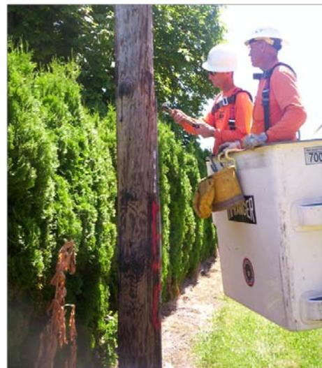
Figure III-10. Line personnel sounding a Douglas-fir transmission pole above the groundline.
