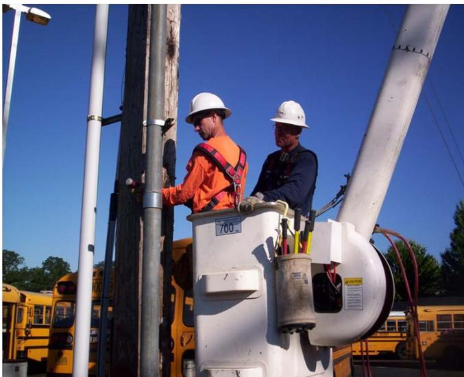
Figure III-9. Line personnel inspecting the above ground zone of a transmission pole.
