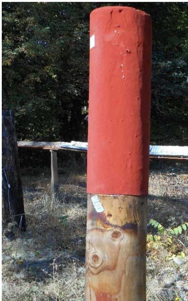
*Figure III-2. Example of a polyurea capped pole top during installation in 2011.*
