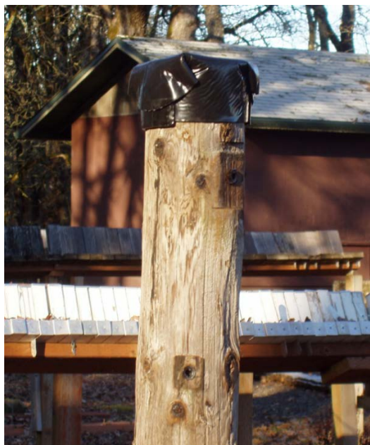
Figure III-19. Example of the condition of water-shedding caps at the start of exposure and after 113 months of exposure in Corvallis, OR.
